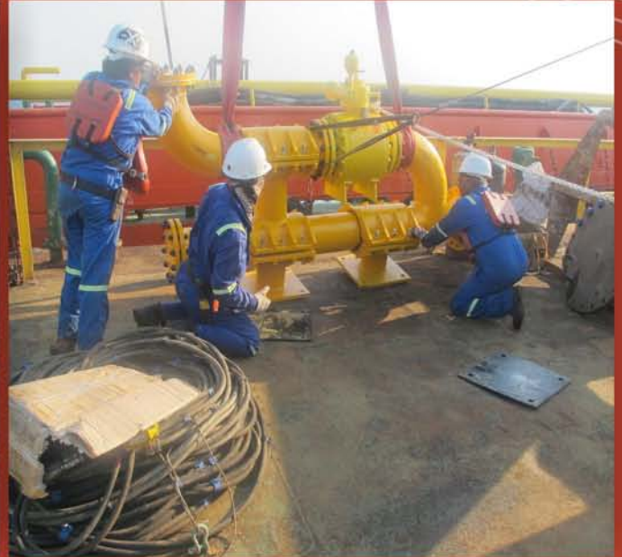
INSTALLATION OF SPOOL PIECE AT PLEM
