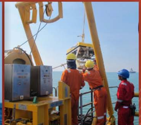
UNDERWATER PIPELINE INSPECTION BY ROV H800 (Poleng Field Madura Offshore, Th. 2013)
