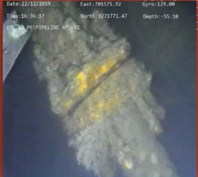
UNDER WATER PIPELINE INSPECTION
