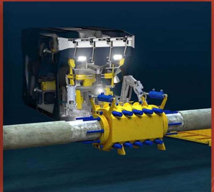
PLIDCO CLAMP INSTALLATION BY ROV WORK CLASS
