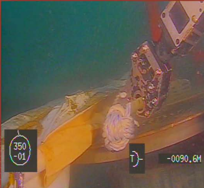
GROUT BAG INSTALLATION
