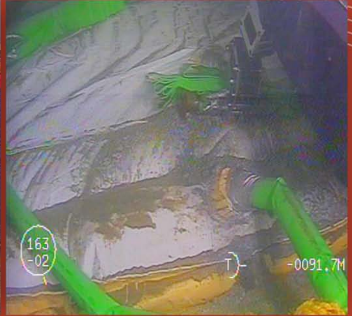
GROUT BAG CEMENT PUMPING
