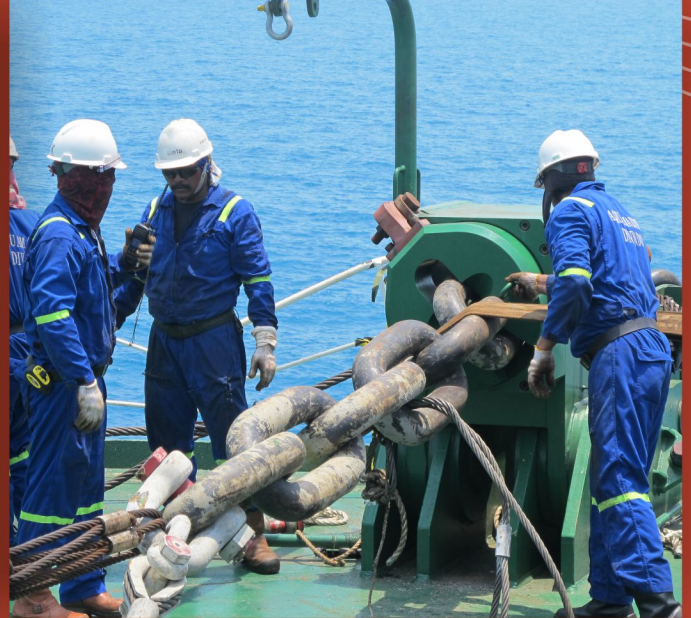
INSTALL CHAIN TO CHAIN STOPPER
