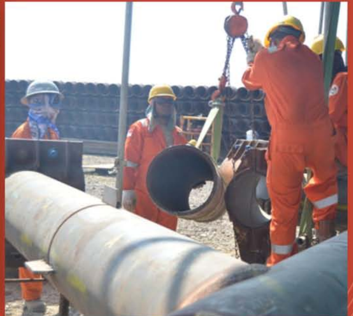
WELDING JOINT CONDUCTOR PIPE
