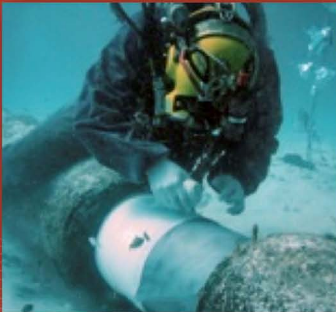
PIPELINE CONCRETE REMOVAL FOR NDT TEST
