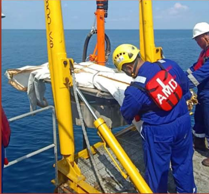
DEPLOYING GROUT BAG TURNTABLE
